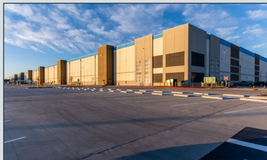
1301 Chalk Hill Road, Dallas, TX
