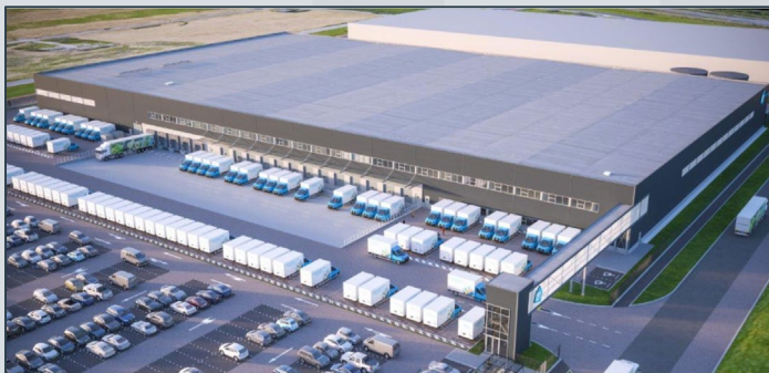
Ahold E-commerce Facility, Bleiswijk, Netherlands
