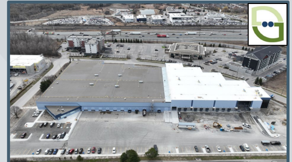
Green Expansion in progress of a building in Ajax, ON, Canada
