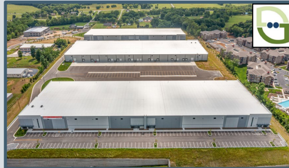
Completed development of three Green Buildings in Lebanon, TN, USA
