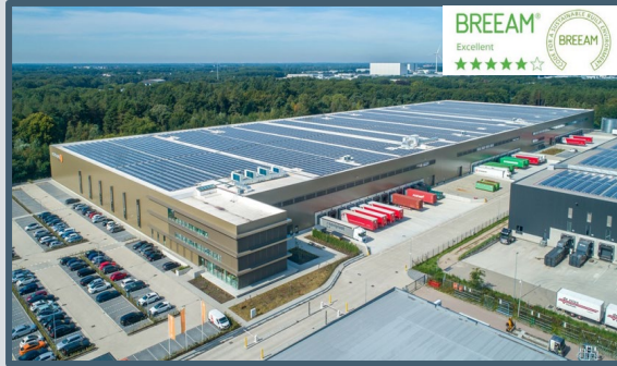
Acquisition and certification (in progress) of a Green Building in Tilburg, Netherlands
